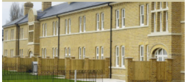
Grade II Heritage conversion of MoD Officers' Mess at the Shoebury Garrison.
